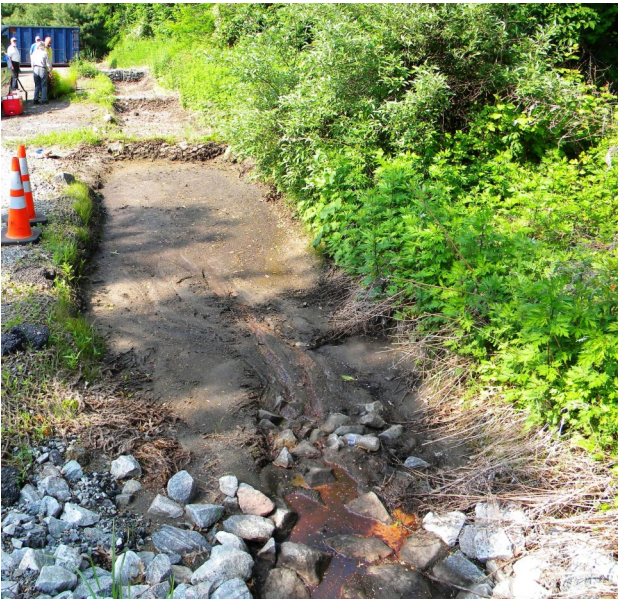
Vegetated swale (1,200 linear feet) with the first cell filled with sediment. Photo credit Pat Rector
