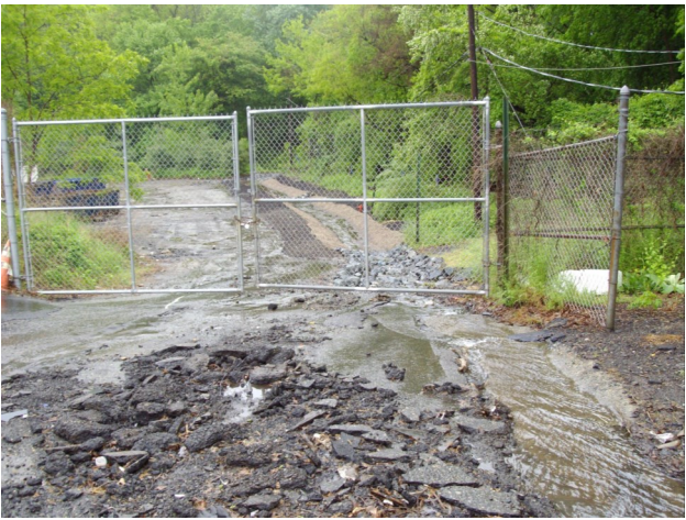
A 66,300 square foot parking lot drains to one area bringing dirt from truck washing and other normal operating dirt along with some residual hydrocarbons from fueling station.
