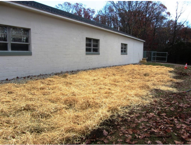
Hay was placed over the excavated garden to maintain the soil and prevent erosion until planting in the spring. Photo credit Jessica Brown. RCE Water Resources Program
